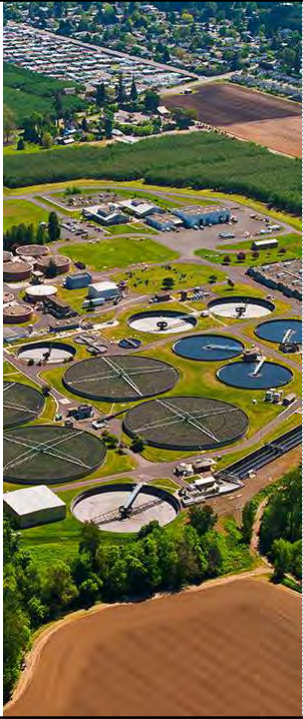
Photo: Willow Lake wastewater recovery facility
