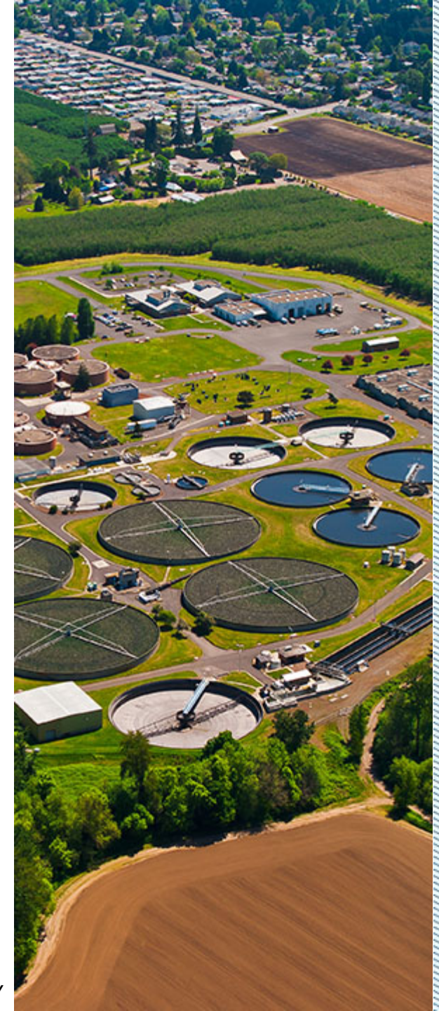
Photo: Willow Lake wastewater recovery facility
