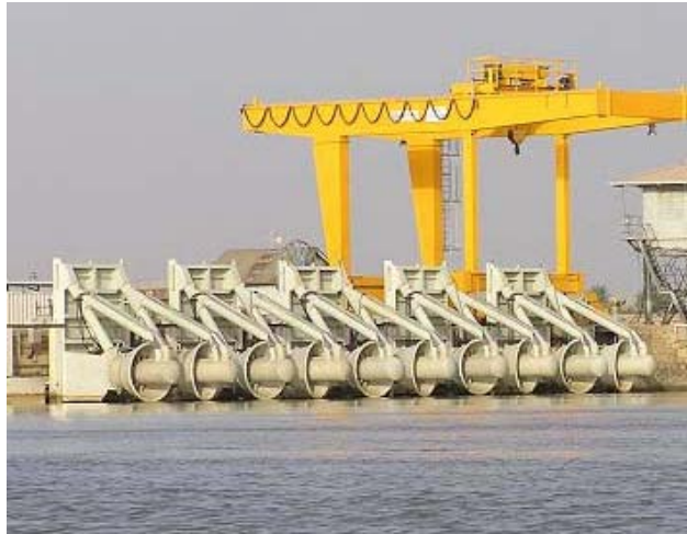
Figure 7. Irrigation dam, Jebel Aulia, Sudan
