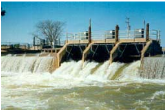
Figure 4. Hydro Installation on the Mulwala Canal, Australia
