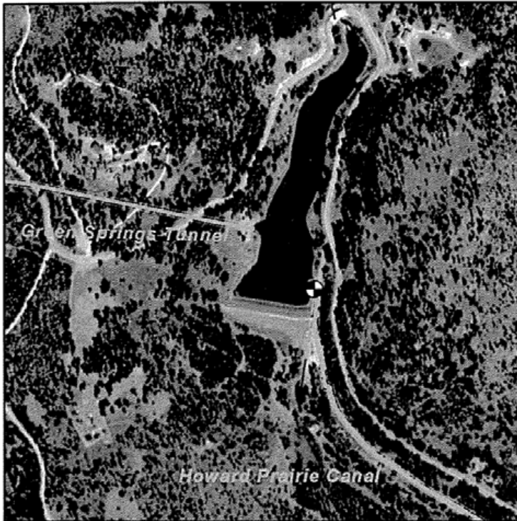
Figure 7: Keene Creek Reservoir power generation site location.
