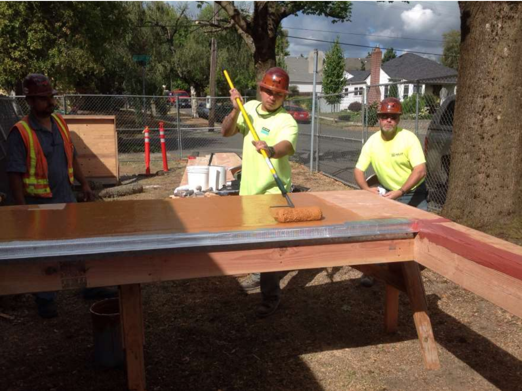
Wall Fabrication And Pre-Application of WRB
