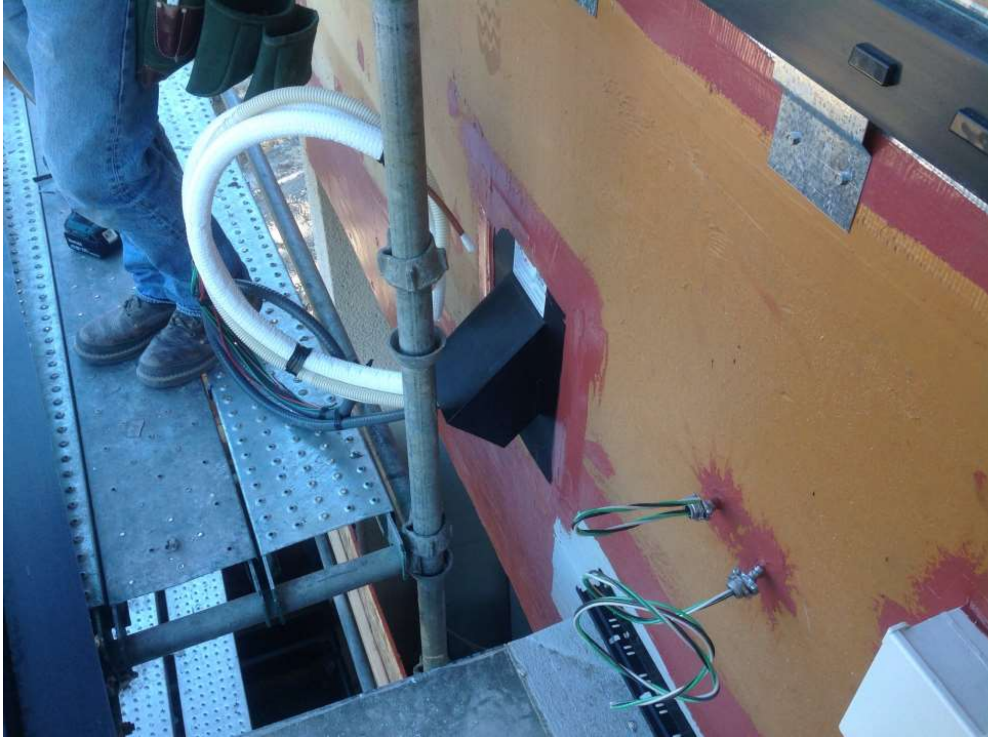
MEP Penetrations Detailed - Ready For Rain-screen Cladding Cover
