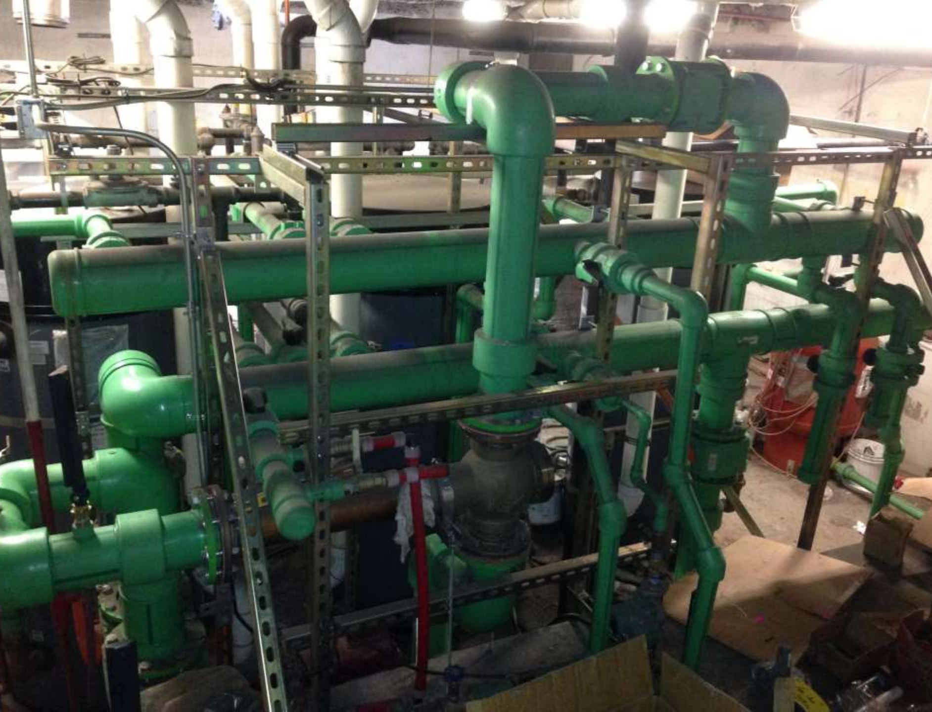
Main Dom Boiler Header Assembly
