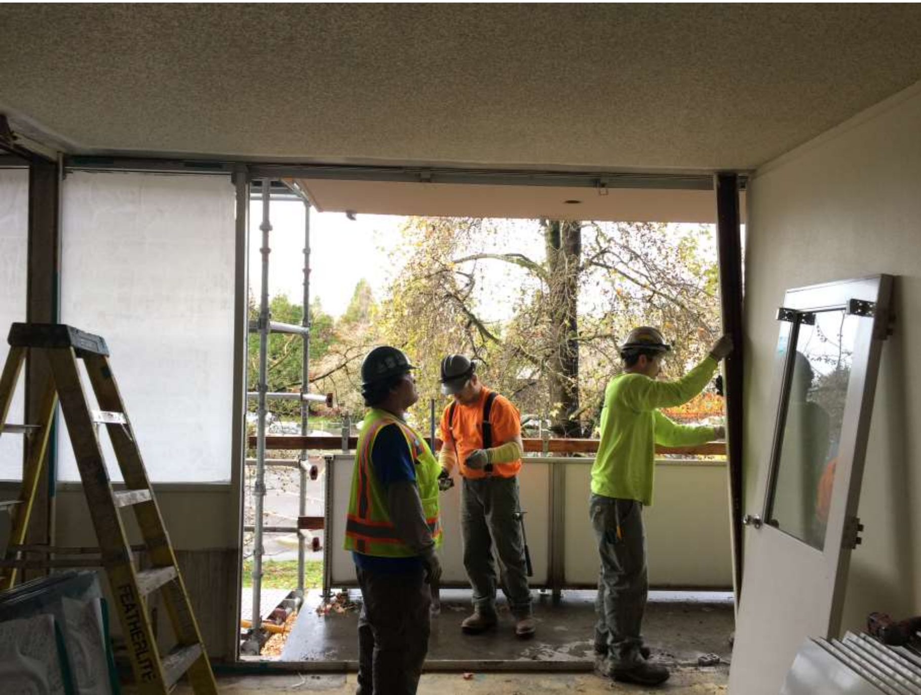
Wall Demo and Abatement of Existing Exterior Components
