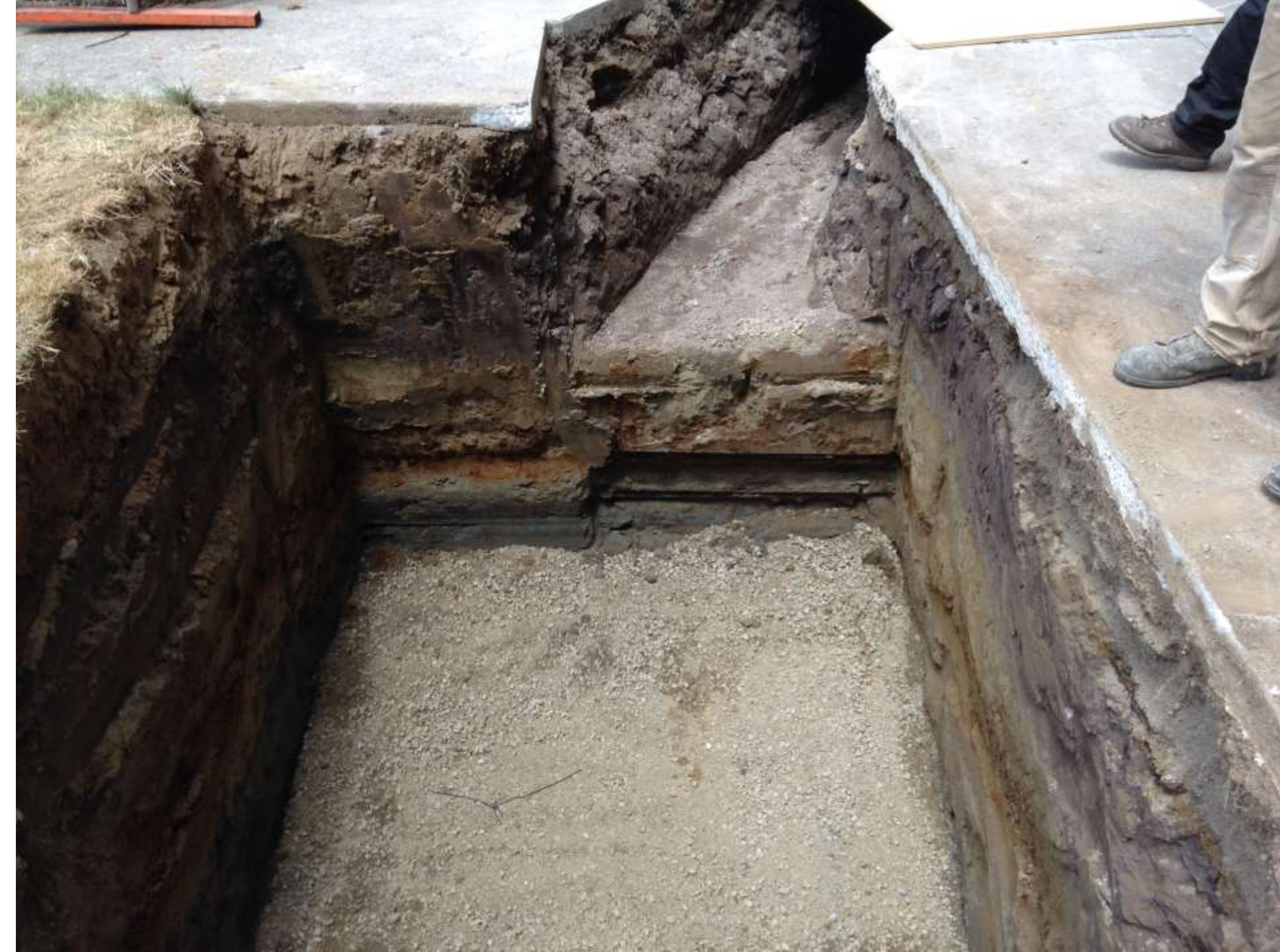
New Dom Water DCVA (Double- Check) Vault Prep
