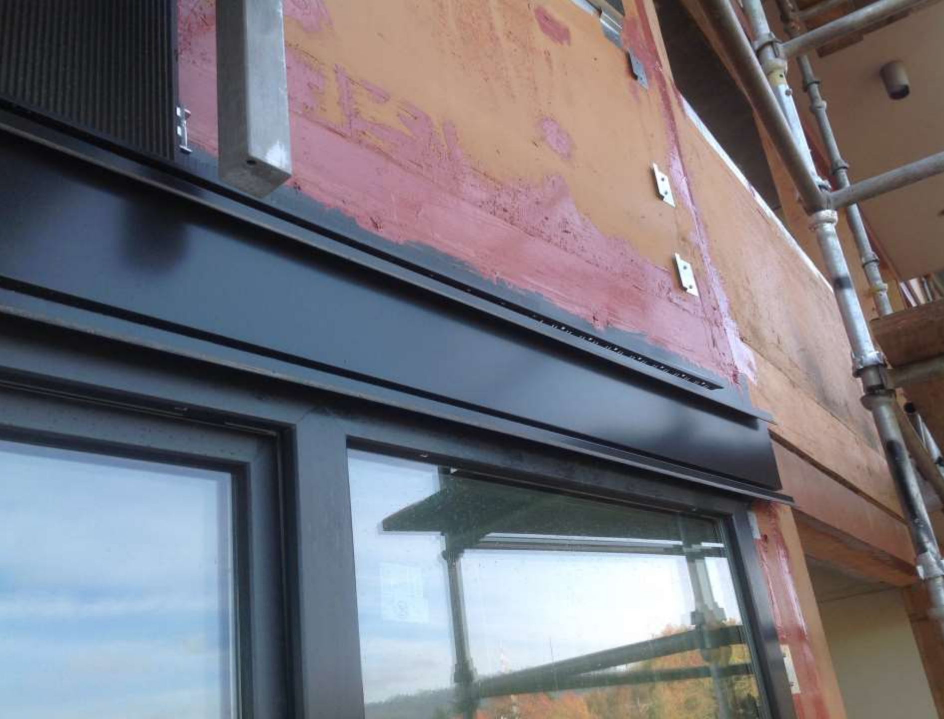
Initial horizontal flashings and clips installed
