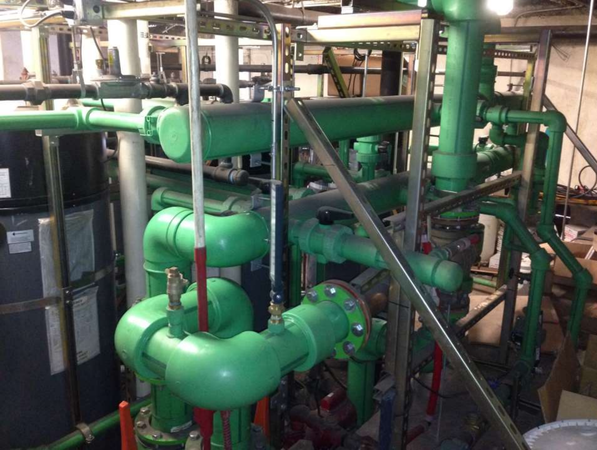
Main Dom Boiler Header Assembly
