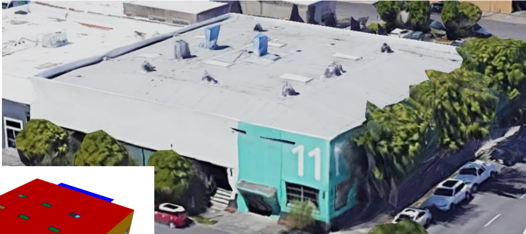
Single Story Existing Office, Portland OR
