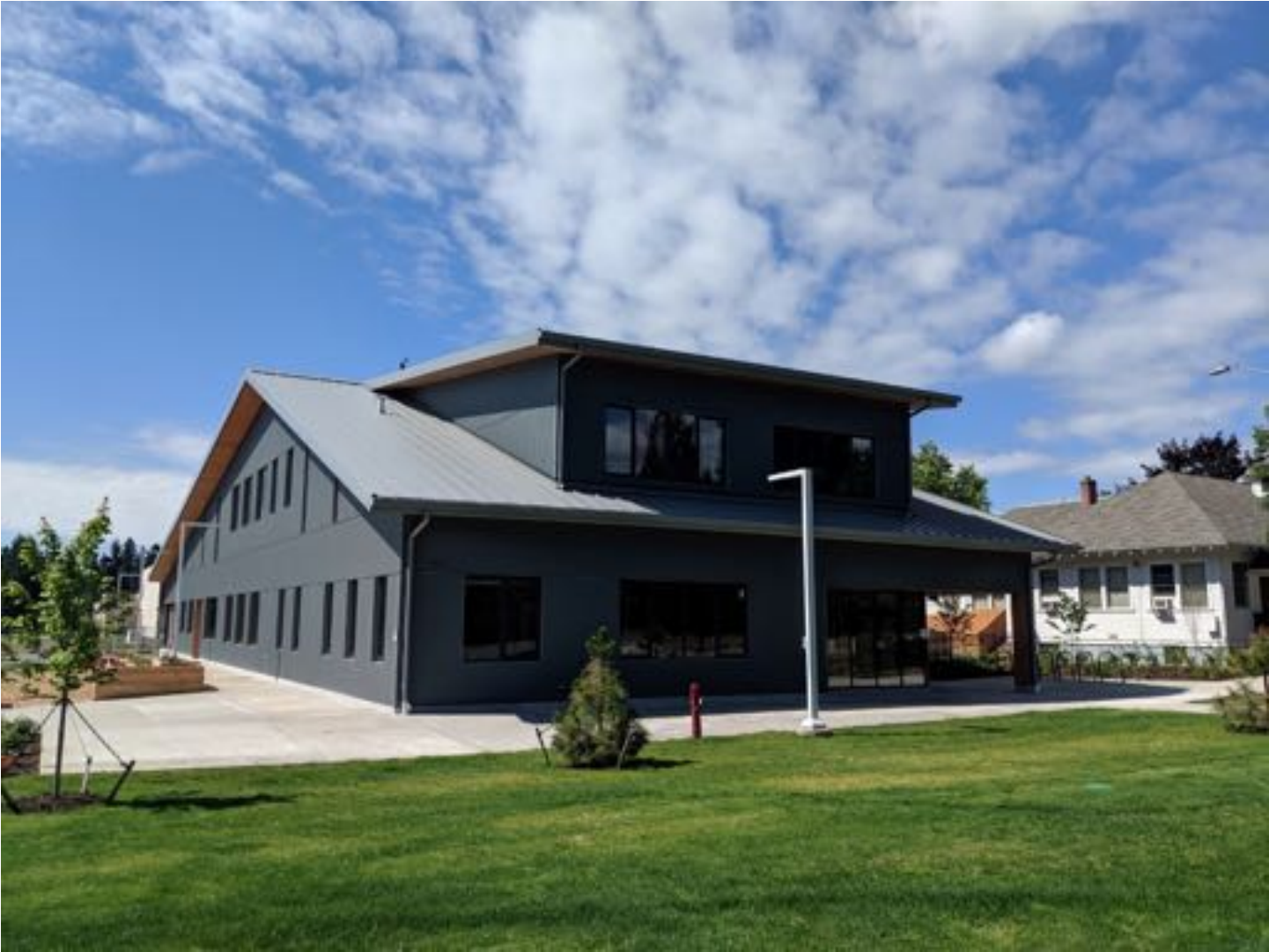
View from North - East
