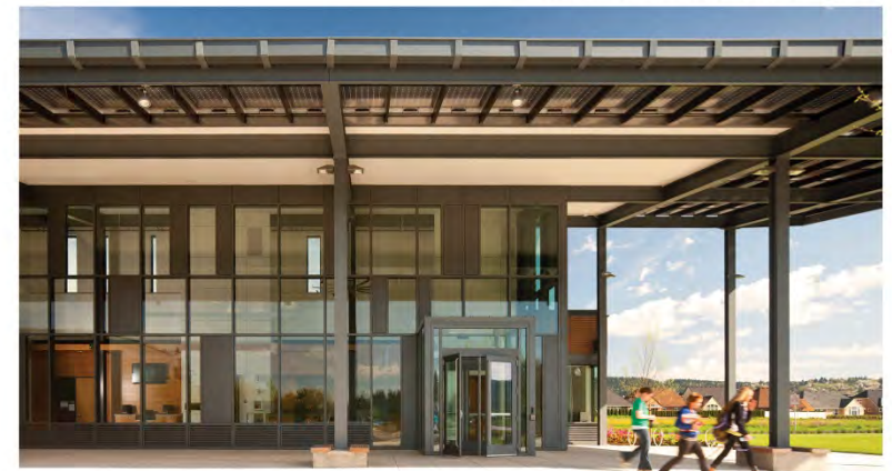
Portland Community College Newberg Center: achieving goals by industry standards
