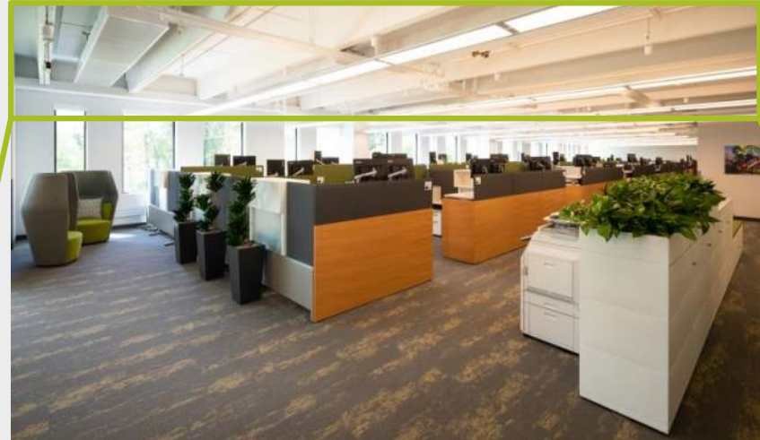
SAIF (Chilled Beam)
