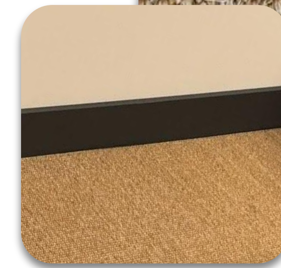
Wood wall base painted to match existing
