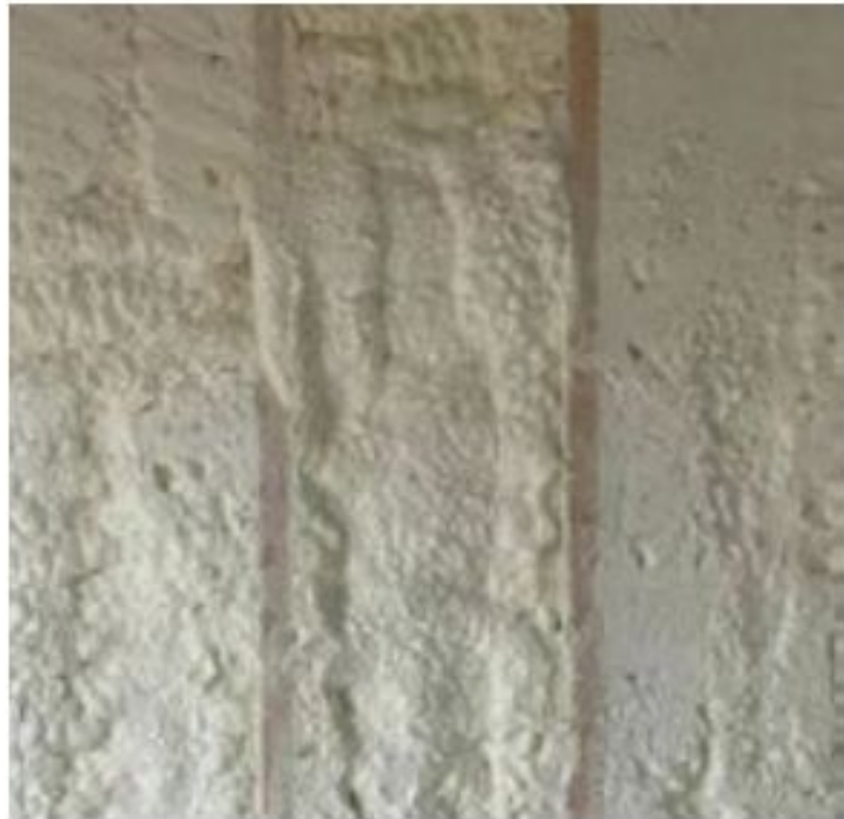
Open Cell Spray Polyurethane Foam
